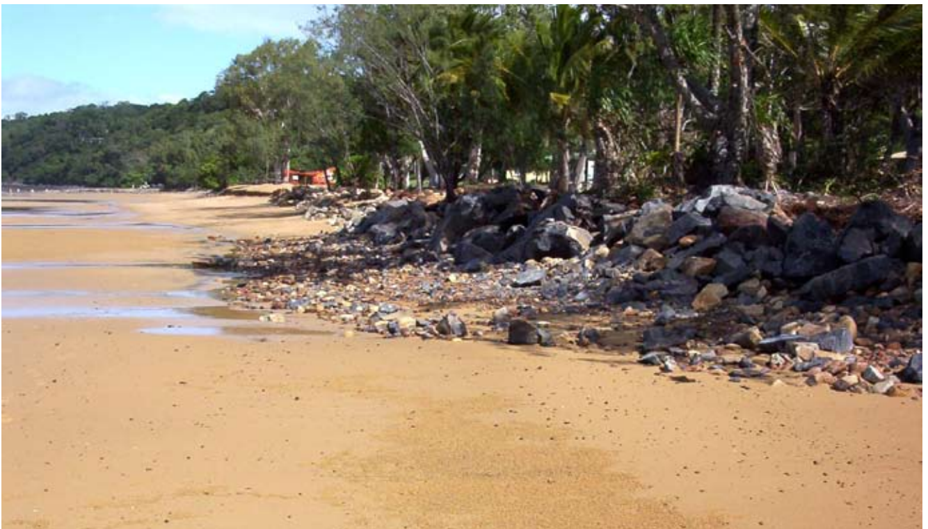
Photo 2. Poorly constructed rock wall at the southern end of South Mission Beach. (source: EPA)
