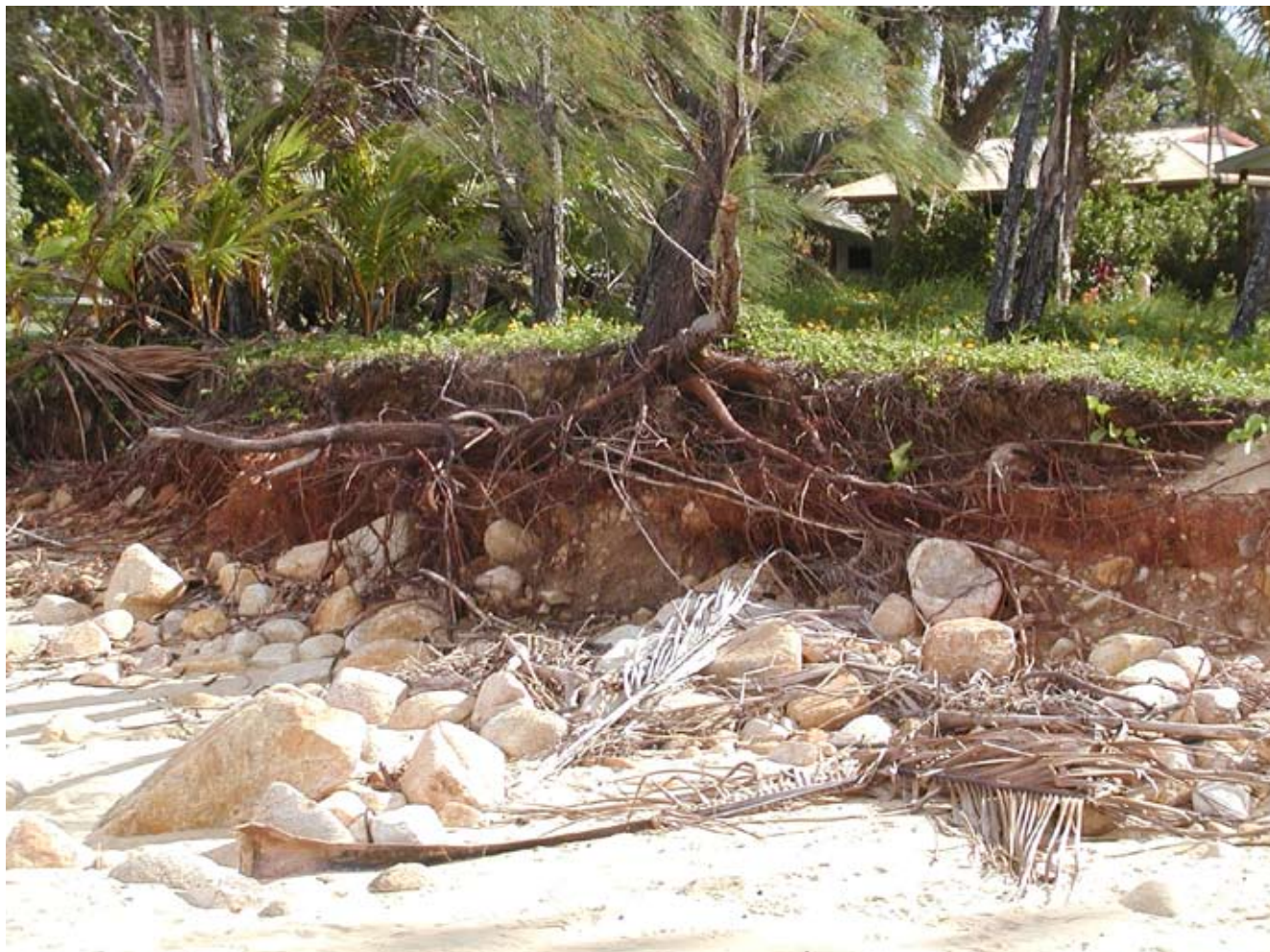
Photo 8. Rock and soil fill material on the esplanade exposed by dune erosion. (source: EPA)
