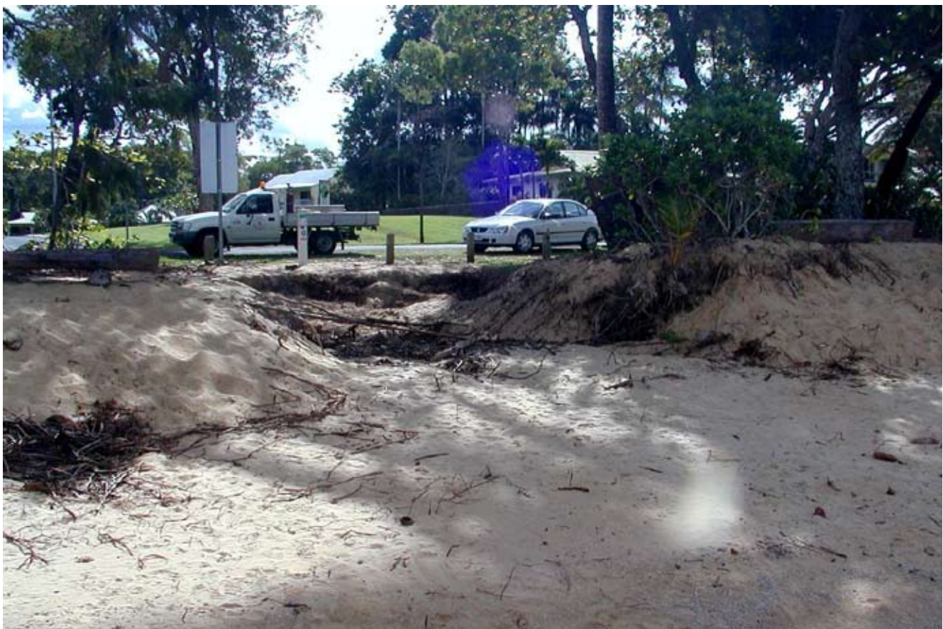
Photo 7. Scour channel through the foredune caused by stormwater overflow, May 2004. (source: EPA)
